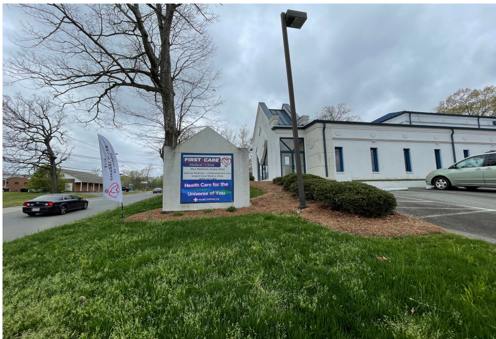
Monument with LED Panel Installed (50 inches high, 75 inches wide)
