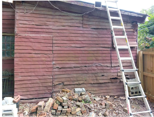
Inappropriate material placed sometime in the 60/70s Which is also failing
