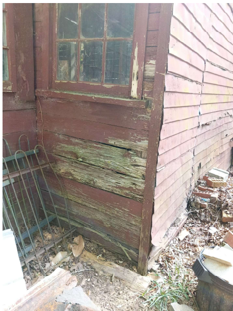
Beasley St view of upper half Wysteria vines have comprised the siding Which allow weather to infiltrate and cause damage
