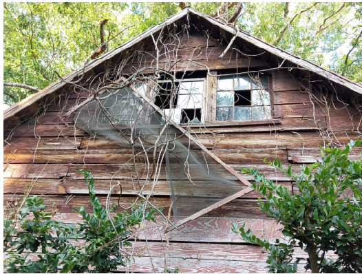
Beasley St view of upper half Wysteria vines have comprised the siding Which allow weather to infiltrate and cause damage
