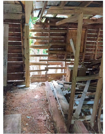
Inside view of photo to the left
