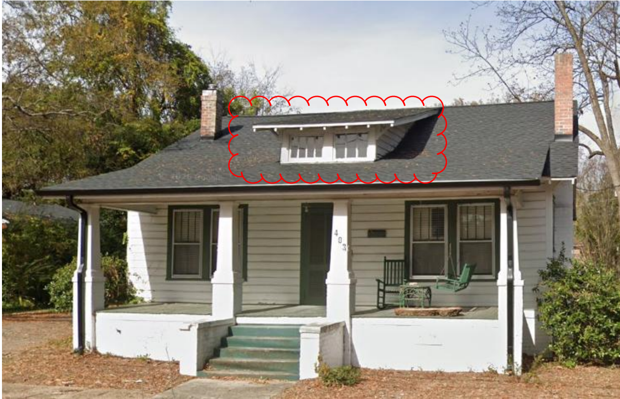
Previous Wood Windows
