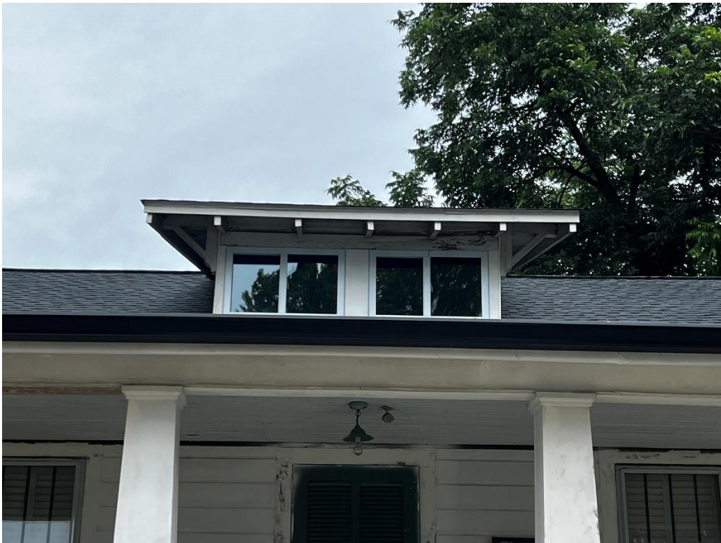
Existing Vinyl Windows
