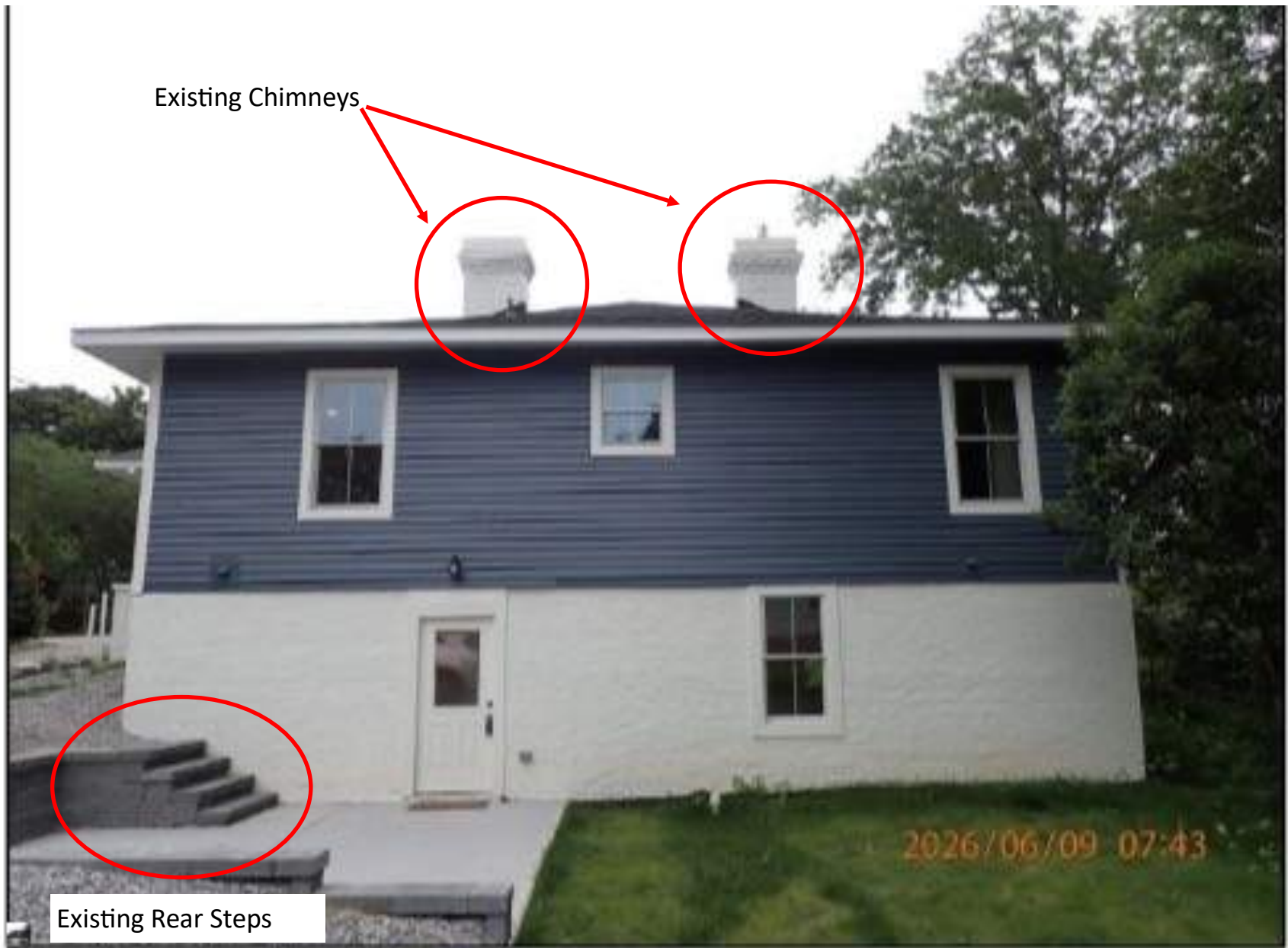
Rear Of Structure
