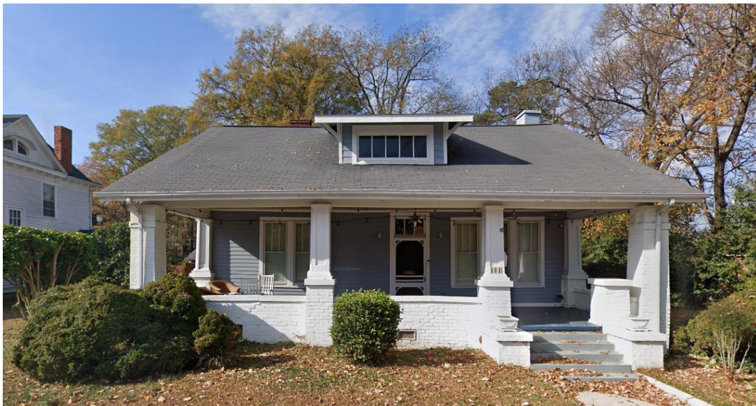
404 South Church Street
