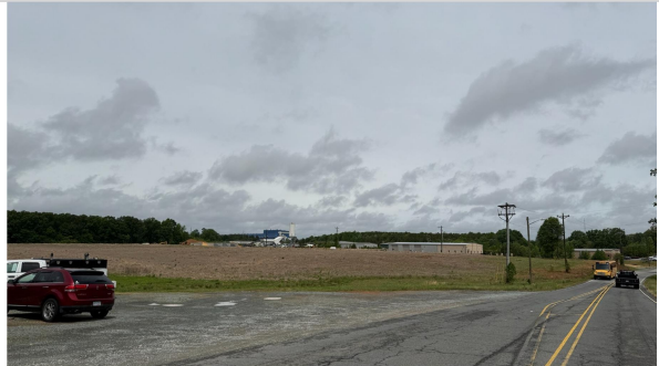
Figure C-6. Existing roadway and corridor conditions adjacent to the subject.
