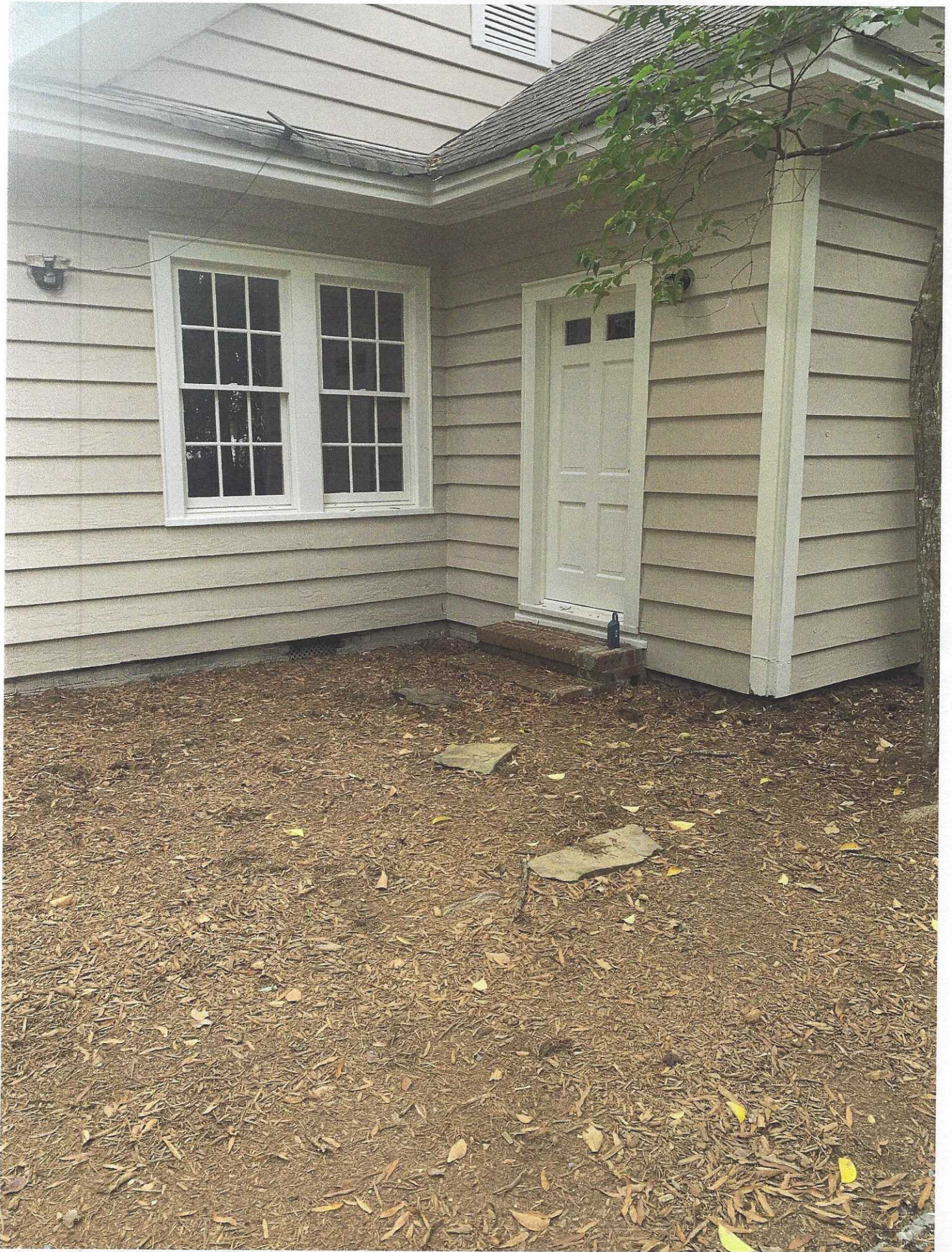
Side entrance where proposed ramp would be placed.
