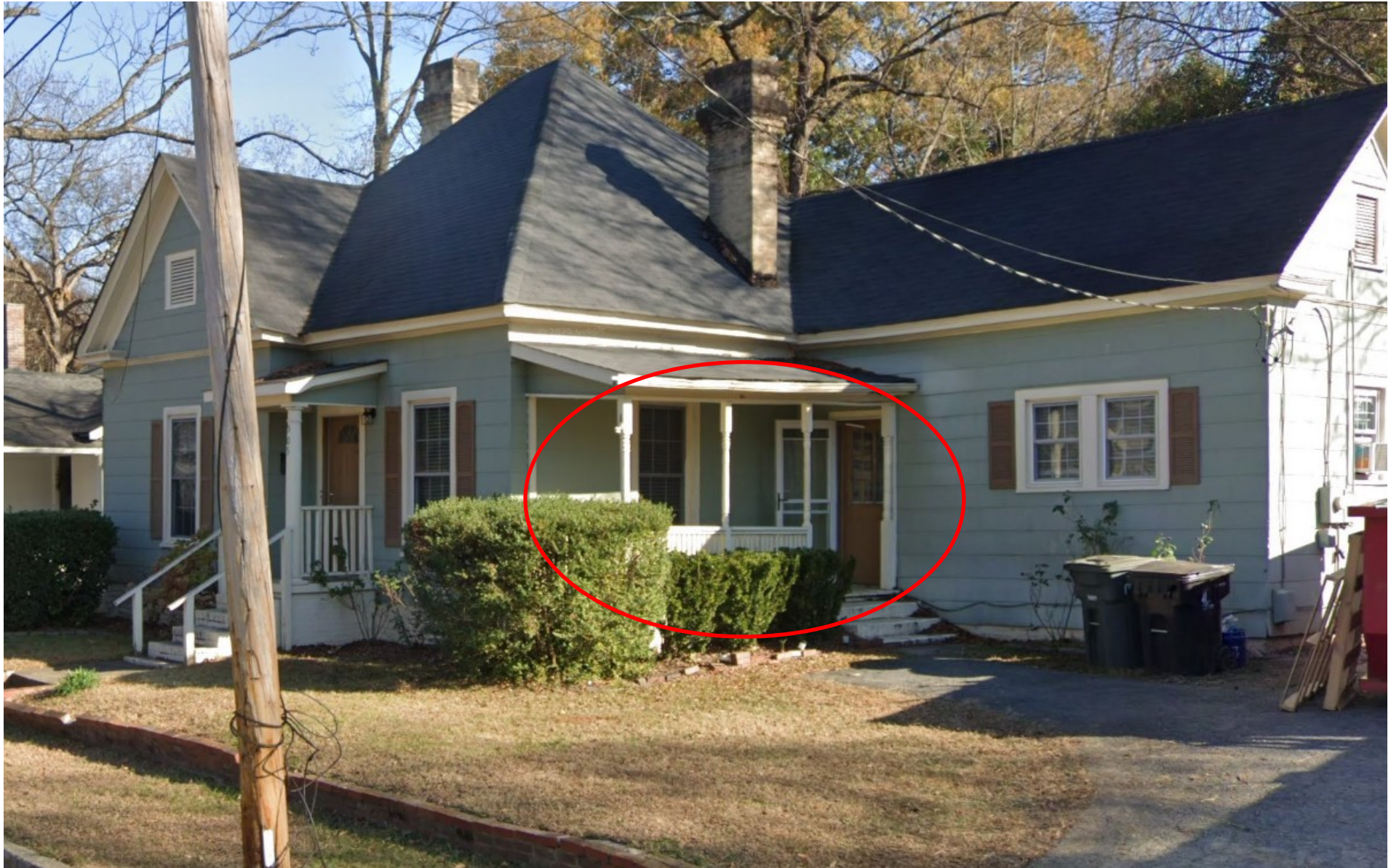
Columns and railing to be removed
