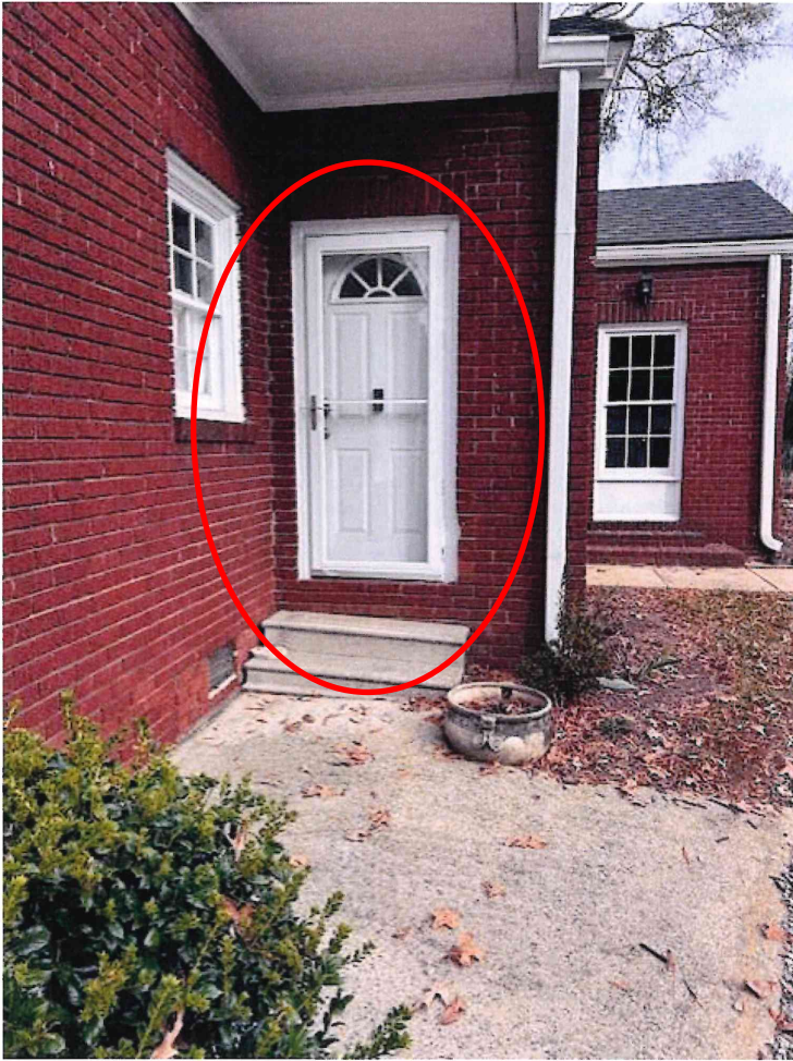
Existing Metal Door to be Replaced
