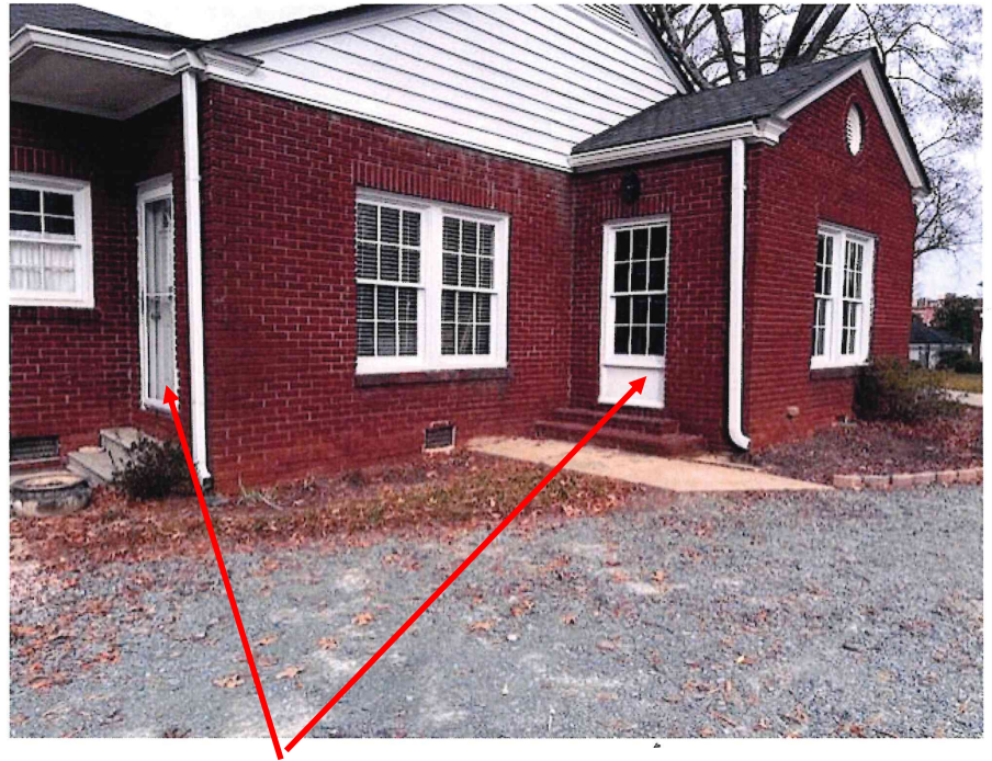
Existing Metal Door to be Replaced. Door and Window Location to be Swapped.
