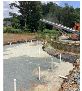
A sand filter in various stages during construction
