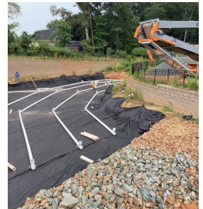
A sand filter in various stages during construction
