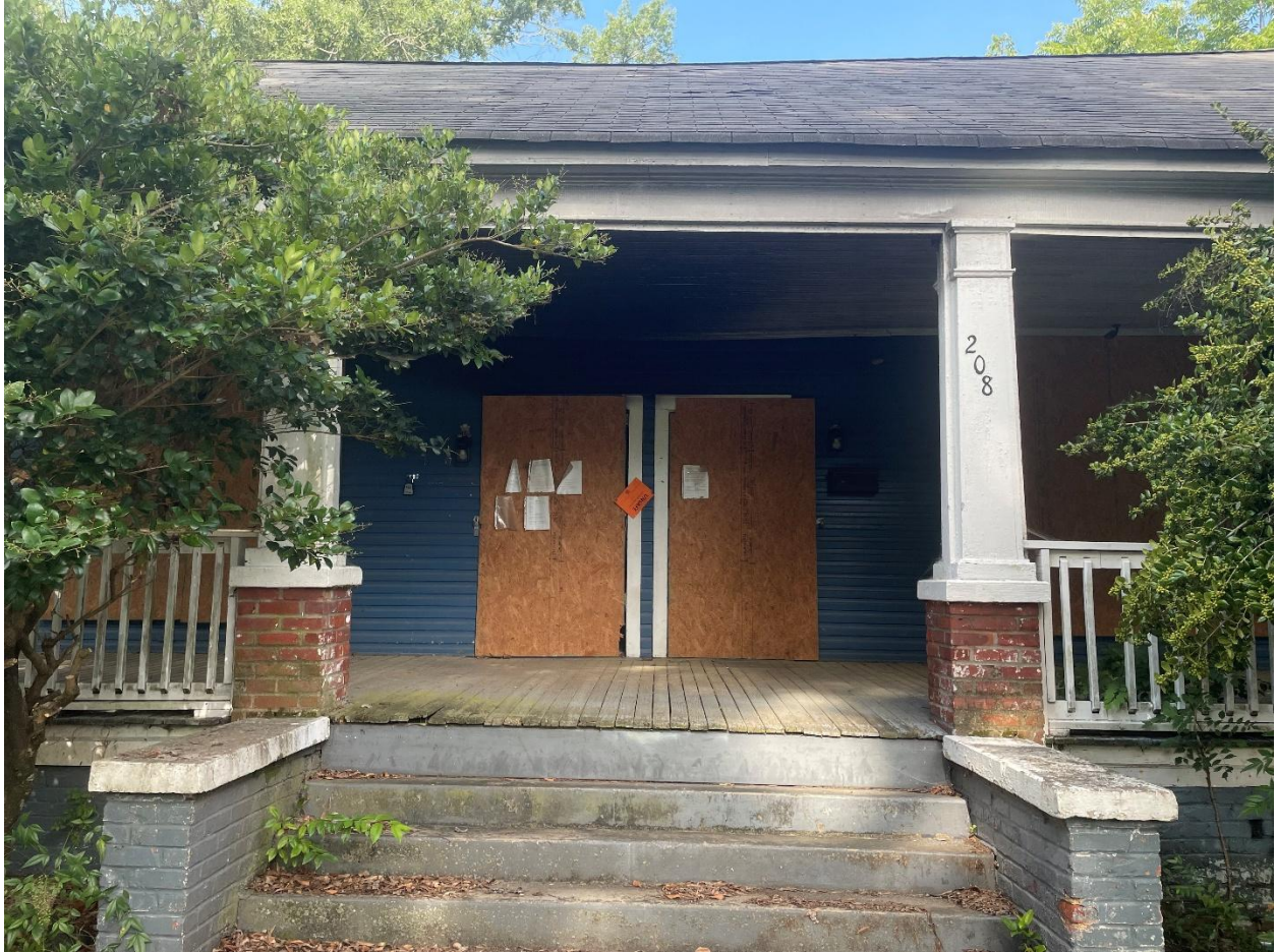
Existing Front Door
