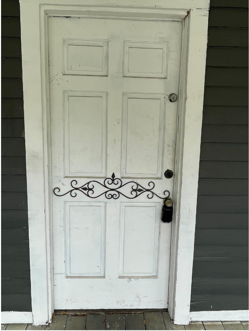
Existing Wood Front Door
