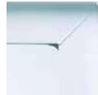
Vinyl sash corner seam
