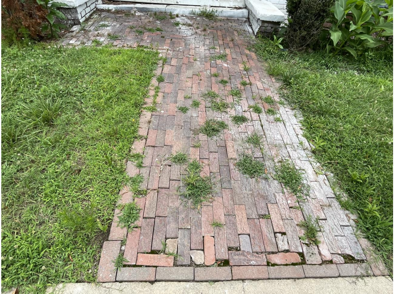
Existing Front Walkway
