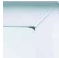
Vinyl sash corner seam
