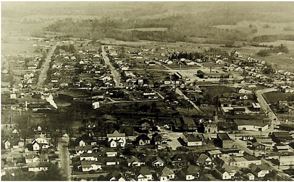
A 1930's view of the roundhouse complex, looking north.
