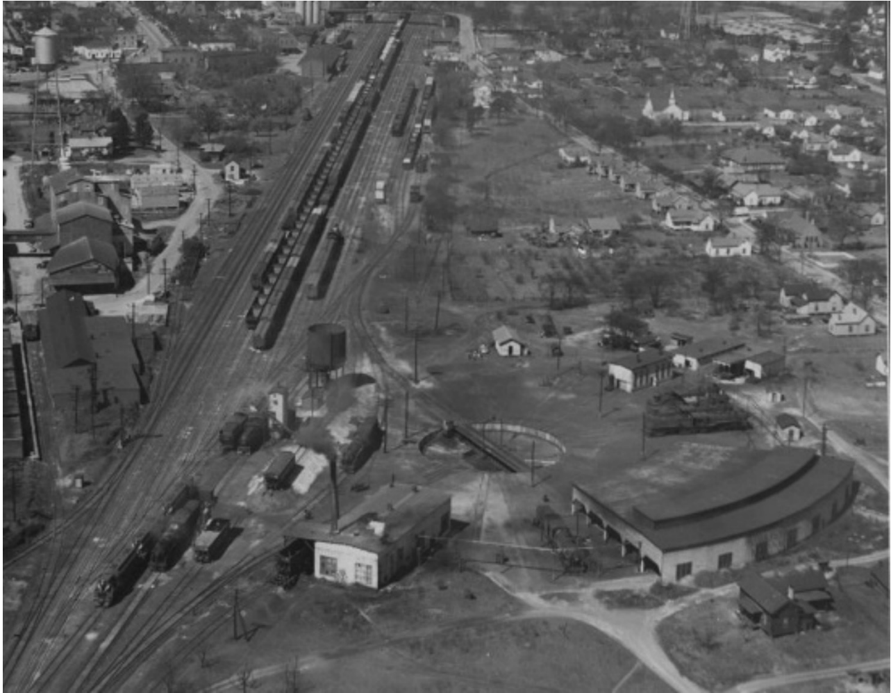
The Seaboard Air Line Railway Company's roundhouse, turntable, sand tower, water tank, oil house, machine shop and office. This aerial photograph was taken c. January 1950, looking west.
