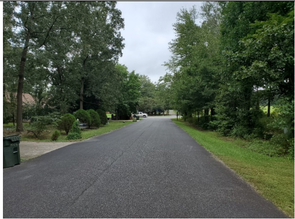
Olde Towne Drive; looking towards Old Charlotte Highway
