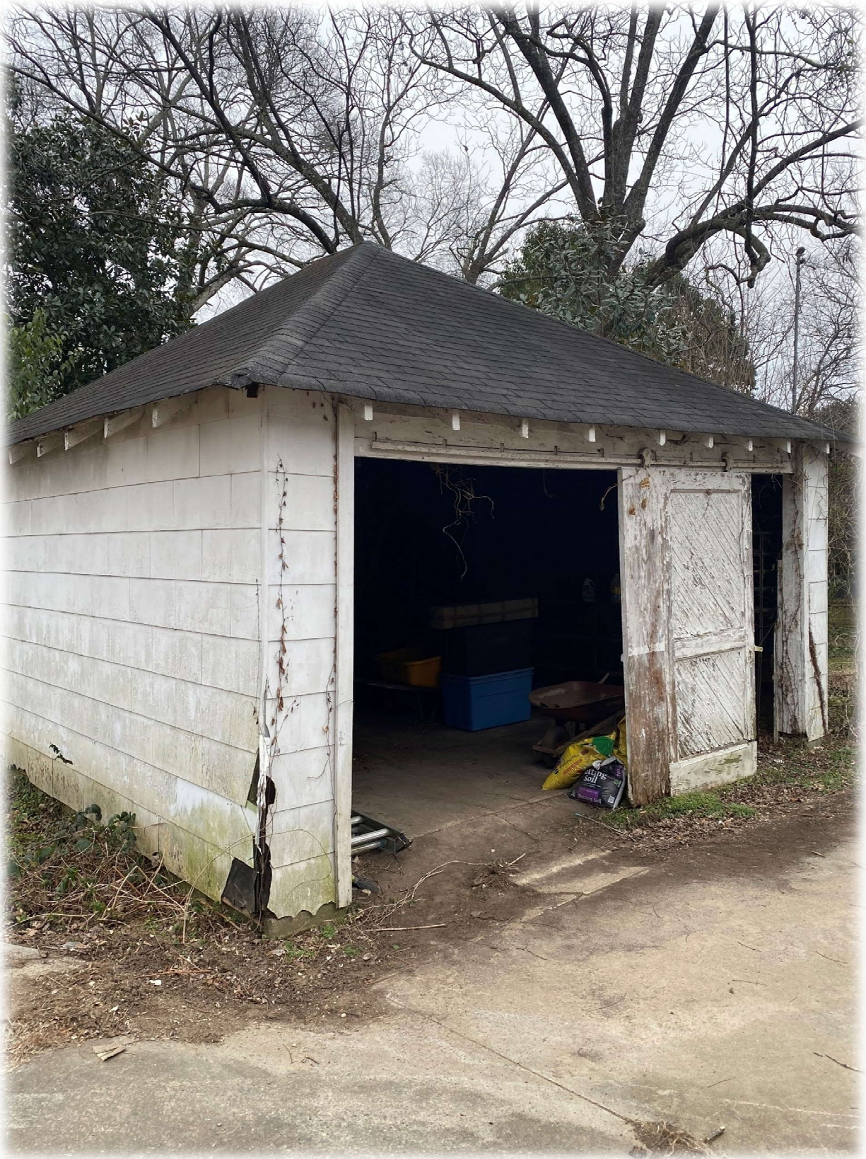
Ex. Garage to be Removed
