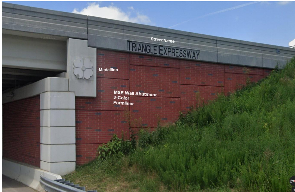
MSE Wall Abutment with 2-Color Form Liner -
