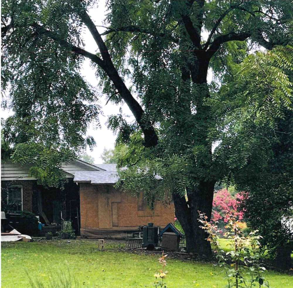
Photo of Violation
