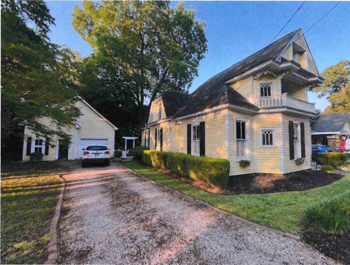
Existing Carriage House and Primary Structure
