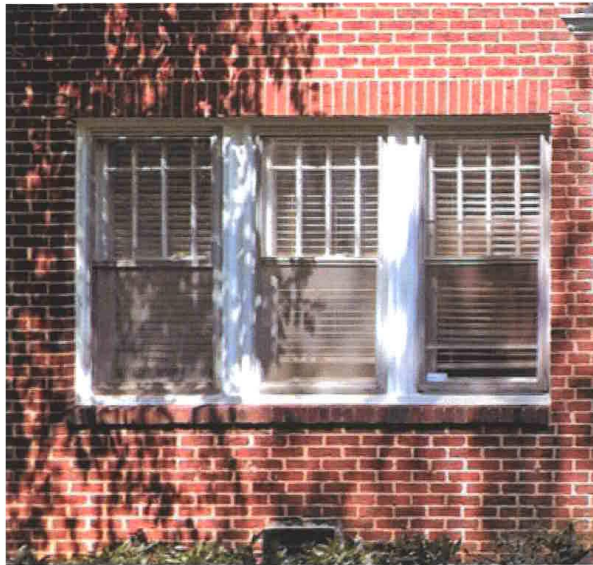
Original Wooden Windows
