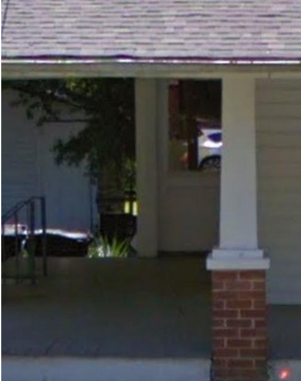
Original Side Front Door
