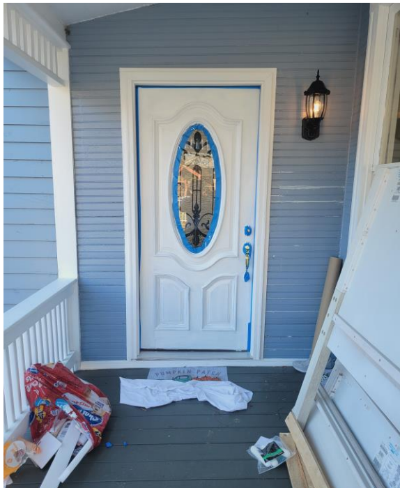
New Door, Painted
