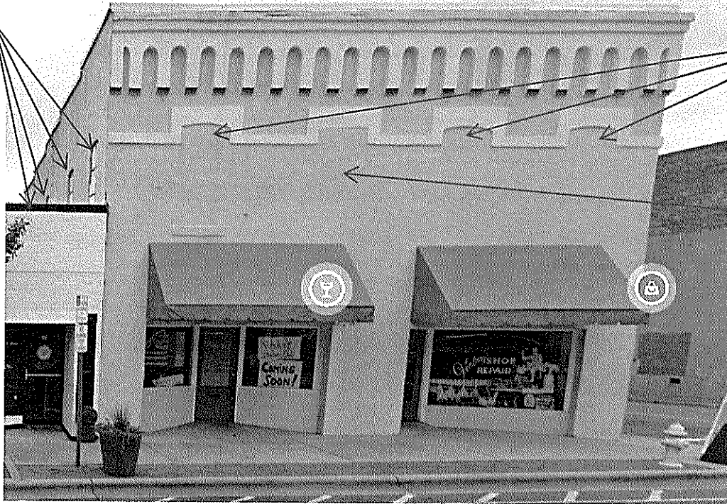
Main St View to front of building
