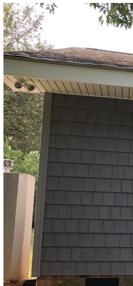
Example of repaired fascia
