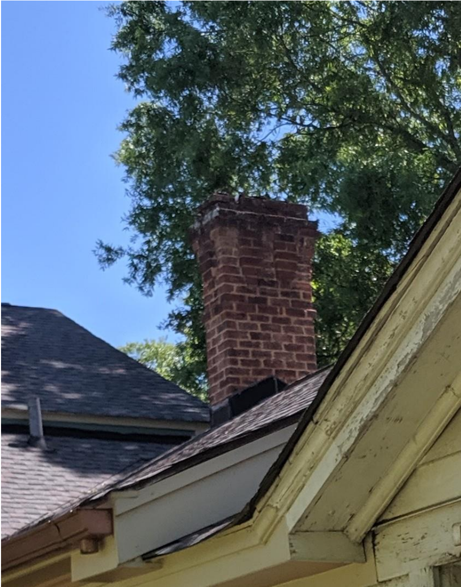
Image of chimney taken up close 4-14-20
