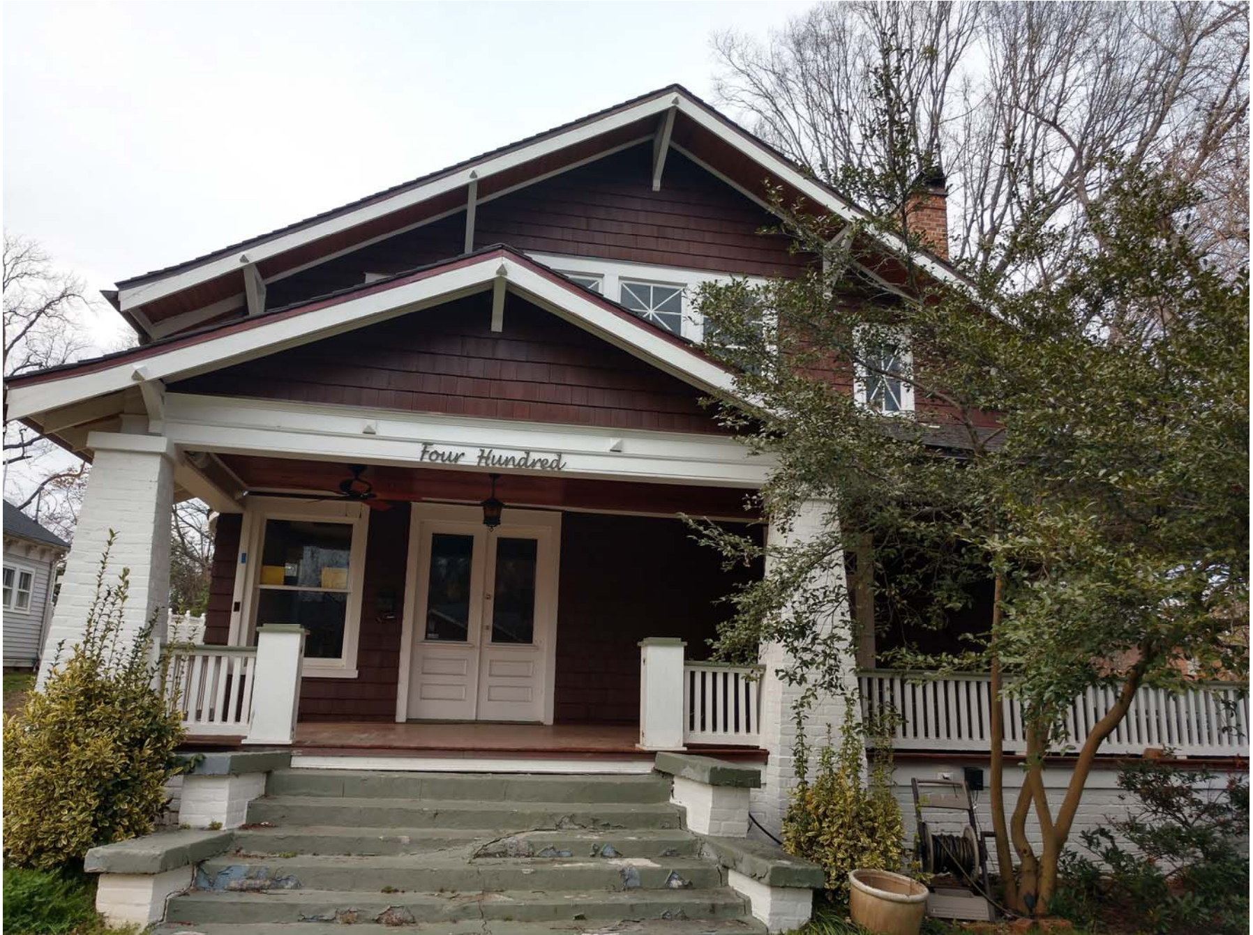
South side— Windsor Street elevation
