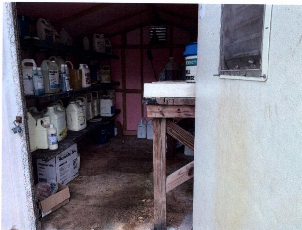
Photograph 7: View pesticide and herbicide storage at Facilities Maintenance without secondary containment.
