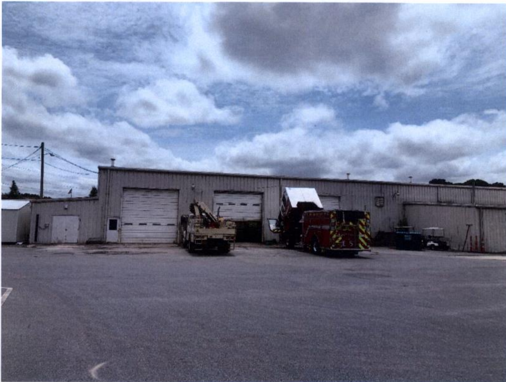
Photograph 2: Additional overview of Monroe Operation Center.
