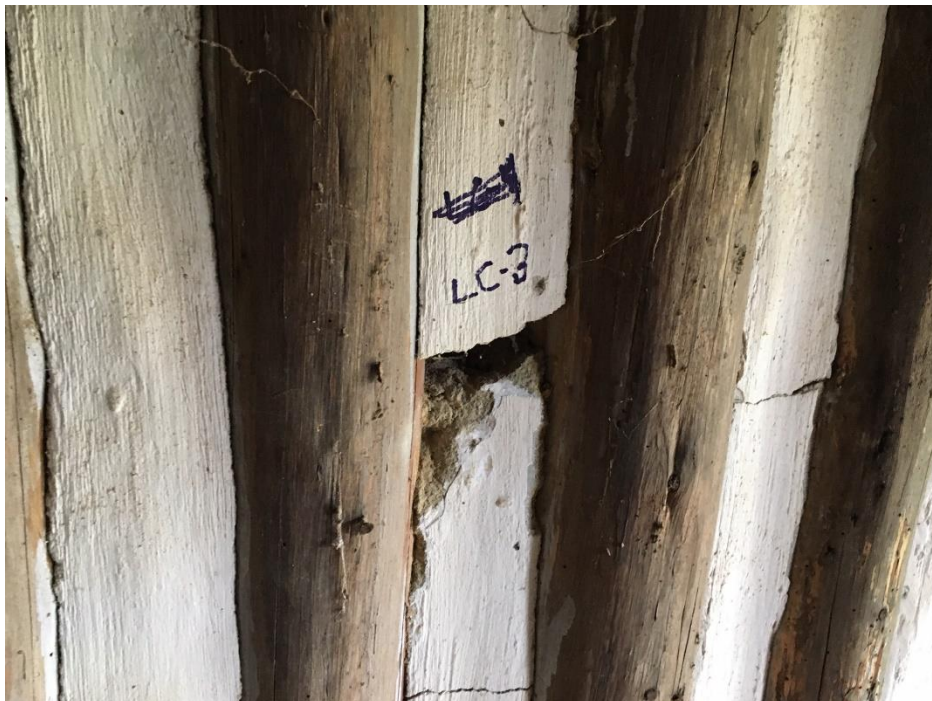
Photo 4 Structure 2 (Parcel 09-301-225B); LC-3 sample location
