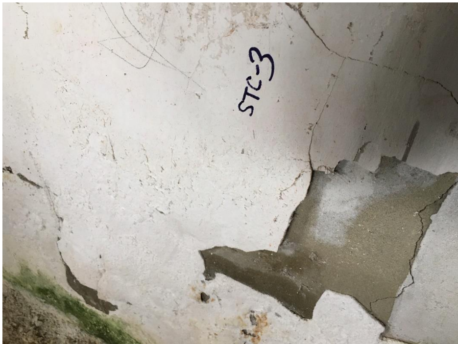
Photo 8 Structure 2 (Parcel 09-301-225B); STC-3 sample location
