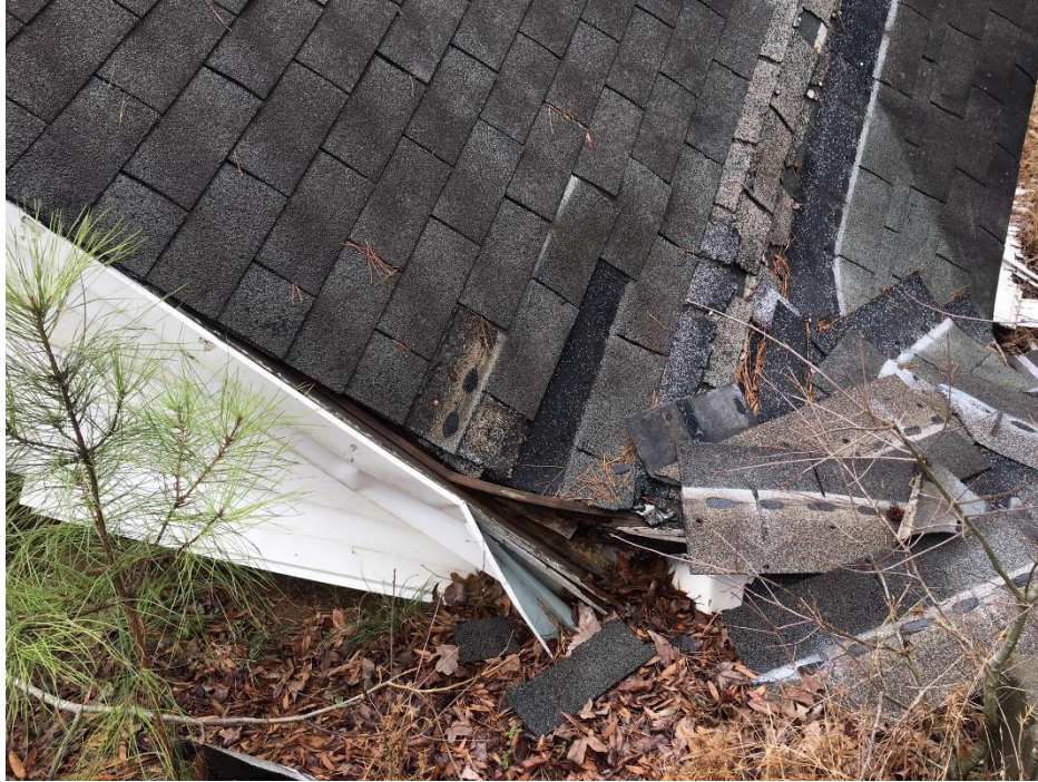
Photo 3 Structure 1; (Parcel 09-301-226B) SHIN-1 through SHIN-6 sample locations
