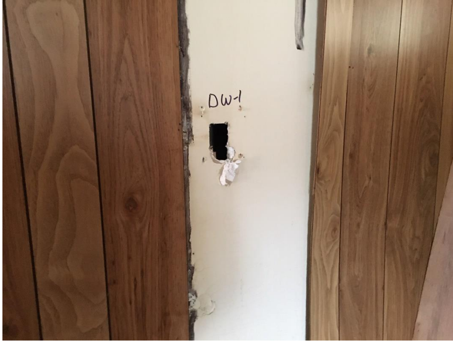
Photo 5 Structure 1; (Parcel 09-301-226B); DW-1 sample location
