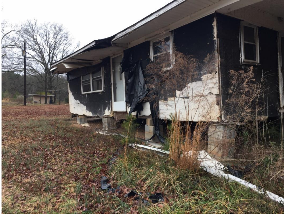
Photo 17 Abandoned structure located on Parcel 09-301-226B
