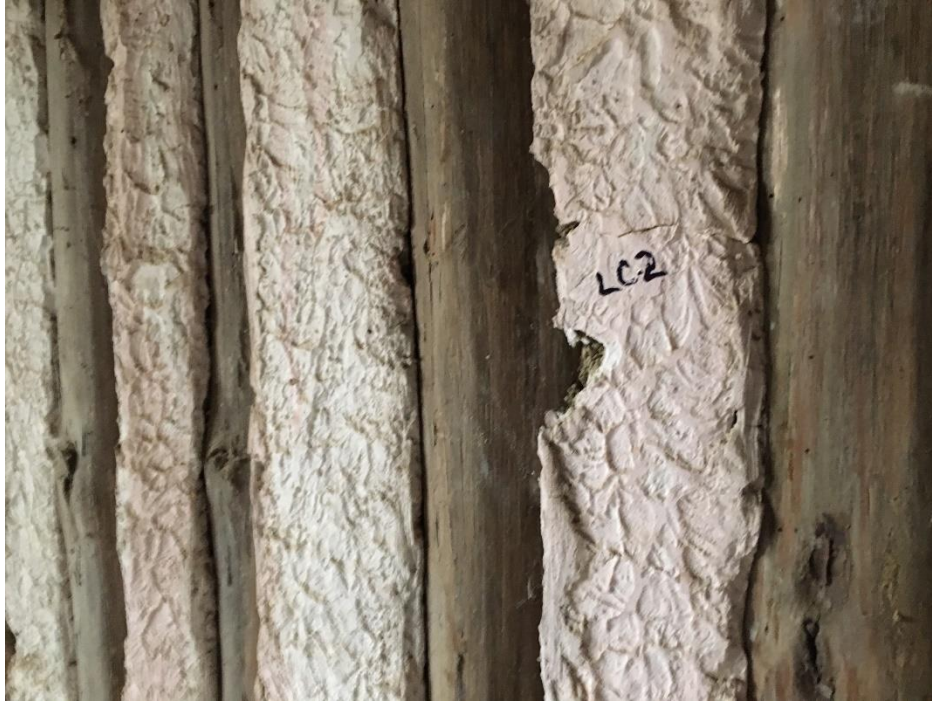
Photo 3 Structure 2 (Parcel 09-301-225B); LC-2 sample location
