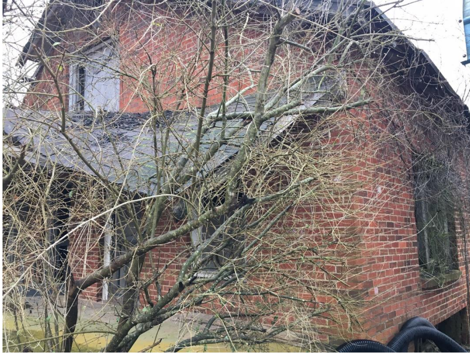
Photo 11 Exterior view of abandoned structure located on Parcel 09-301-225B
