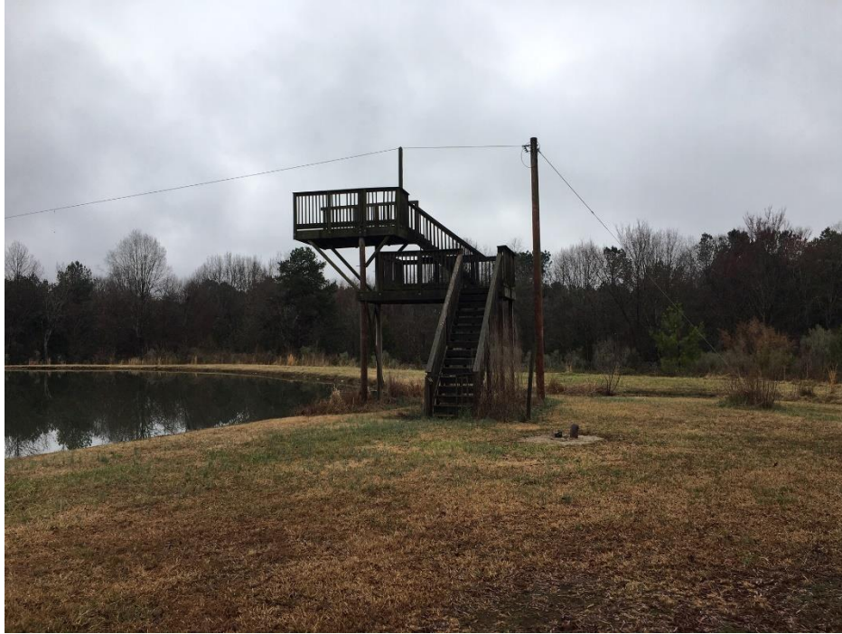
Photo 25 Diving platform located at western end of the pond located on Parcel 09-301-226B
