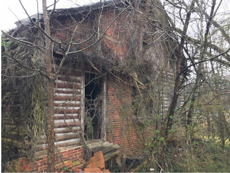
Photo 13 Exterior view of abandoned structure located on Parcel 09-301-225B
