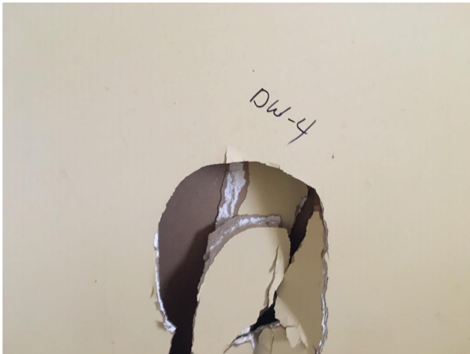
Photo 8 Structure 1; (Parcel 09-301-226B); DW-4 sample location
