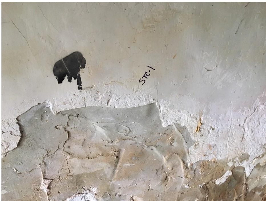
Photo 6 Structure 2 (Parcel 09-301-225B); STC-1 sample location
