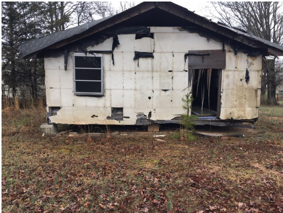
Photo 18 Abandoned structure located on Parcel 09-301-226B
