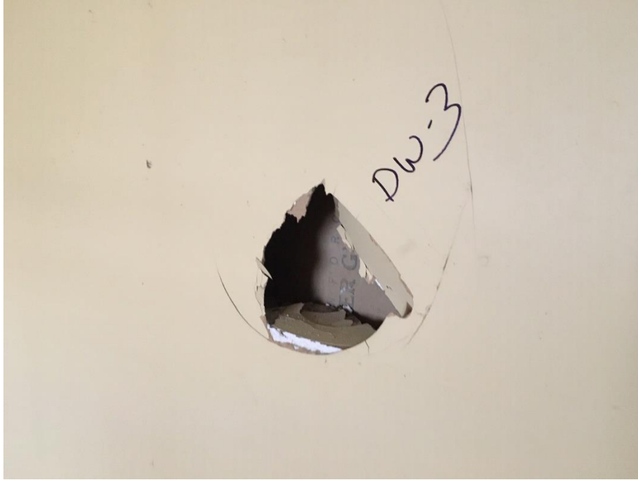
Photo 7 Structure 1; (Parcel 09-301-226B); DW-3 sample location
