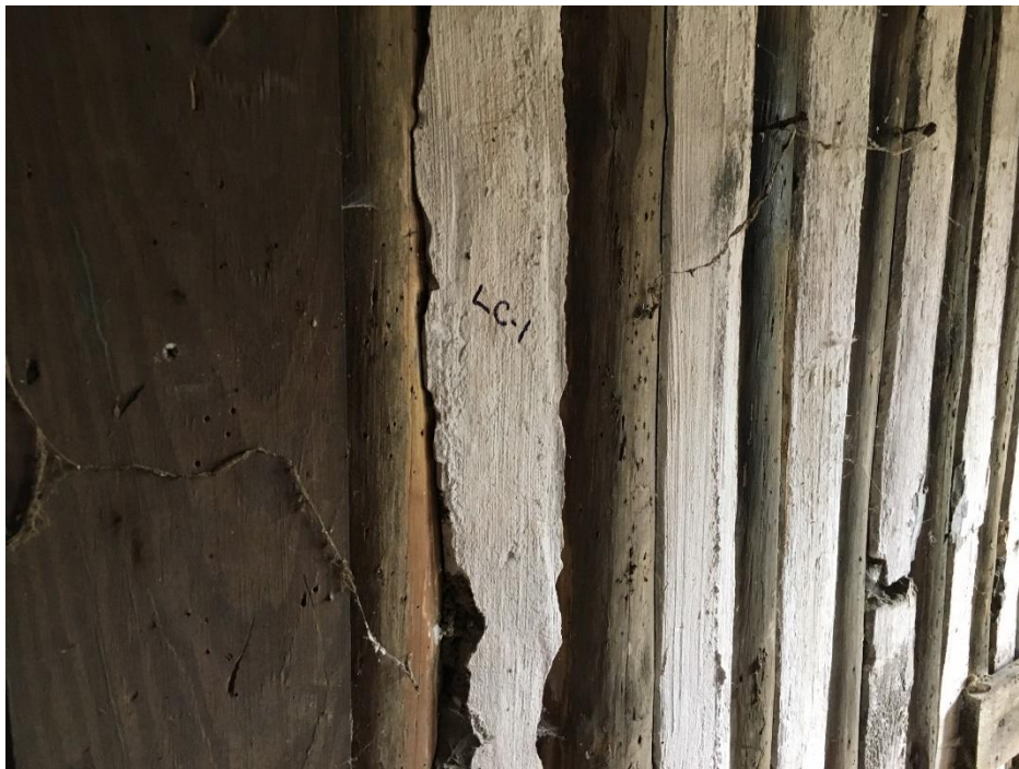
Photo 2 Structure 2 (Parcel 09-301-225B); LC-1 sample location
