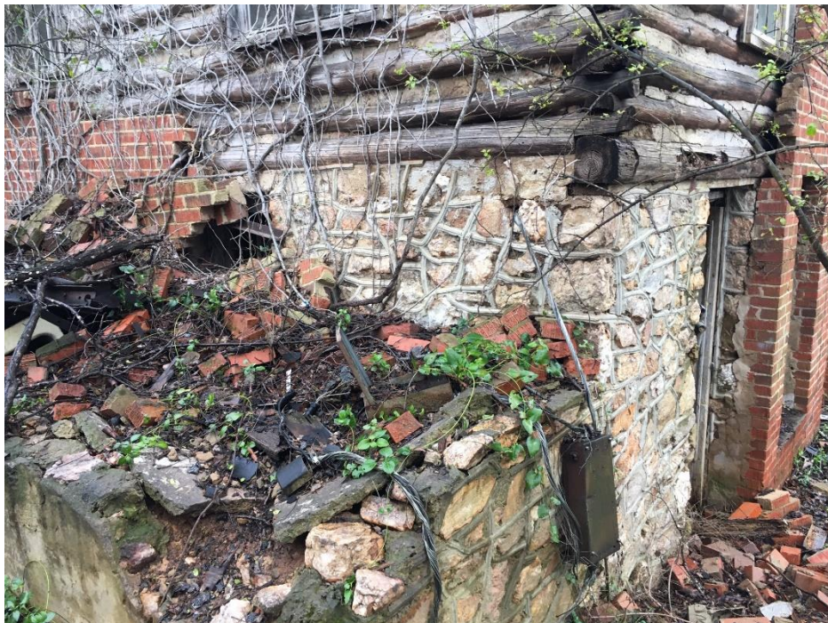
Photo 14 Exterior view of abandoned structure located on Parcel 09-301-225B
