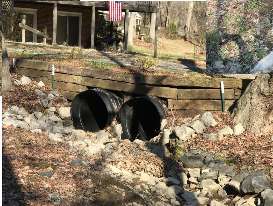
Driveway pipes at 2207 Melody Drive
