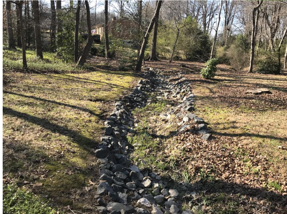
Riprap lined ditch at 2201 Melody Drive
