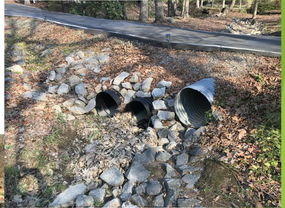
Driveway pipes at 2201 Melody Drive
