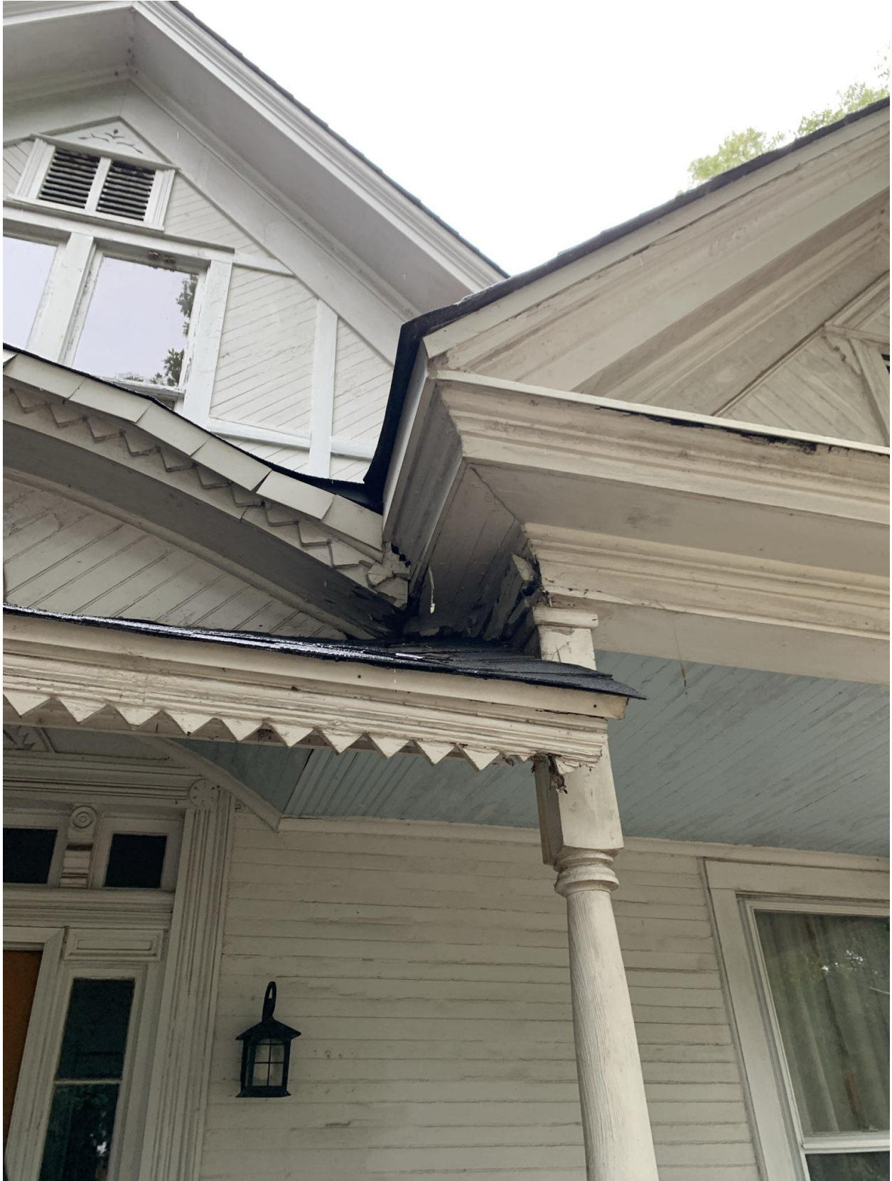
Existing columns on front porch
