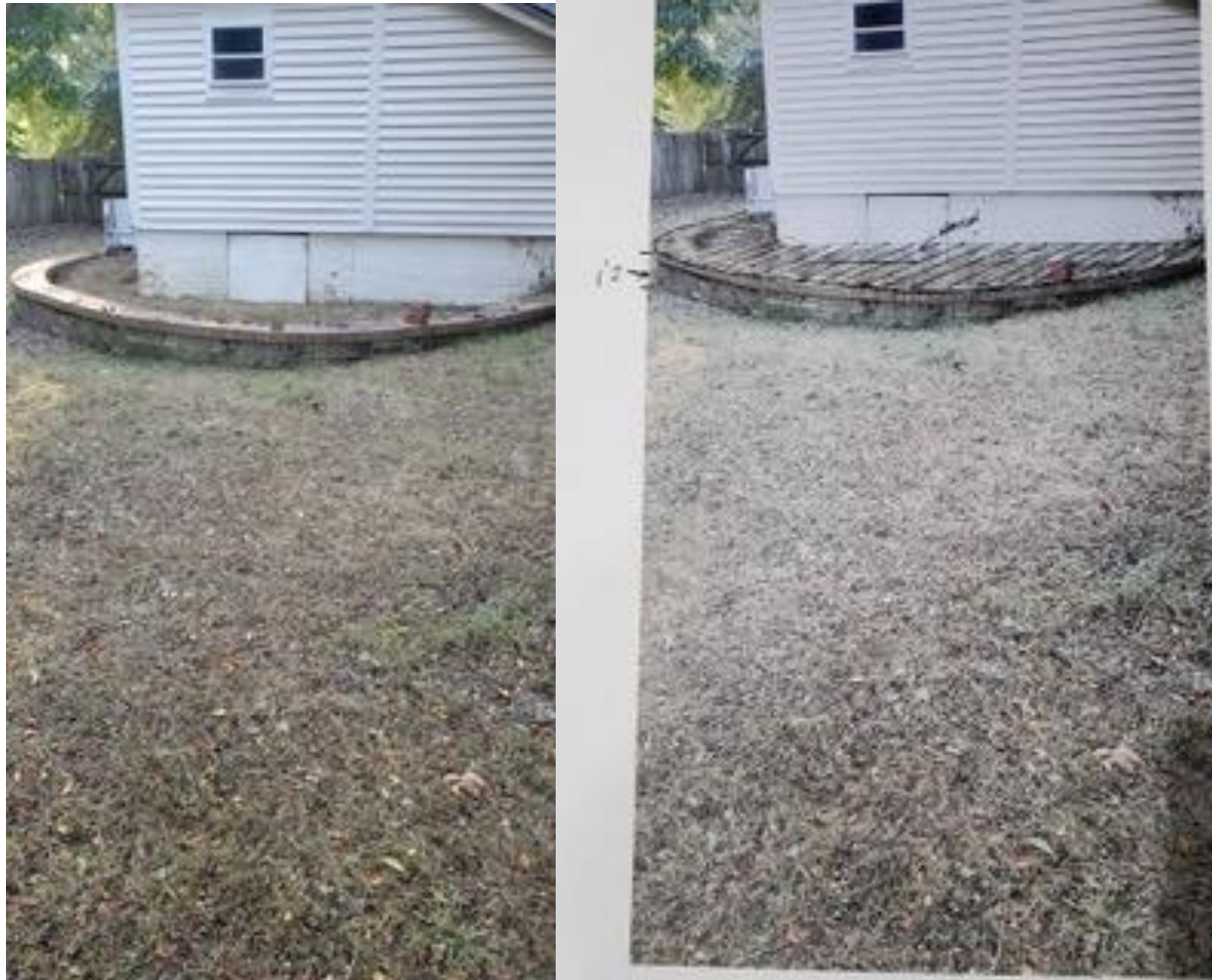
Rear brick oval area - Applicant is proposing to add pressure treated wood decking to this area in the rear of the house.
