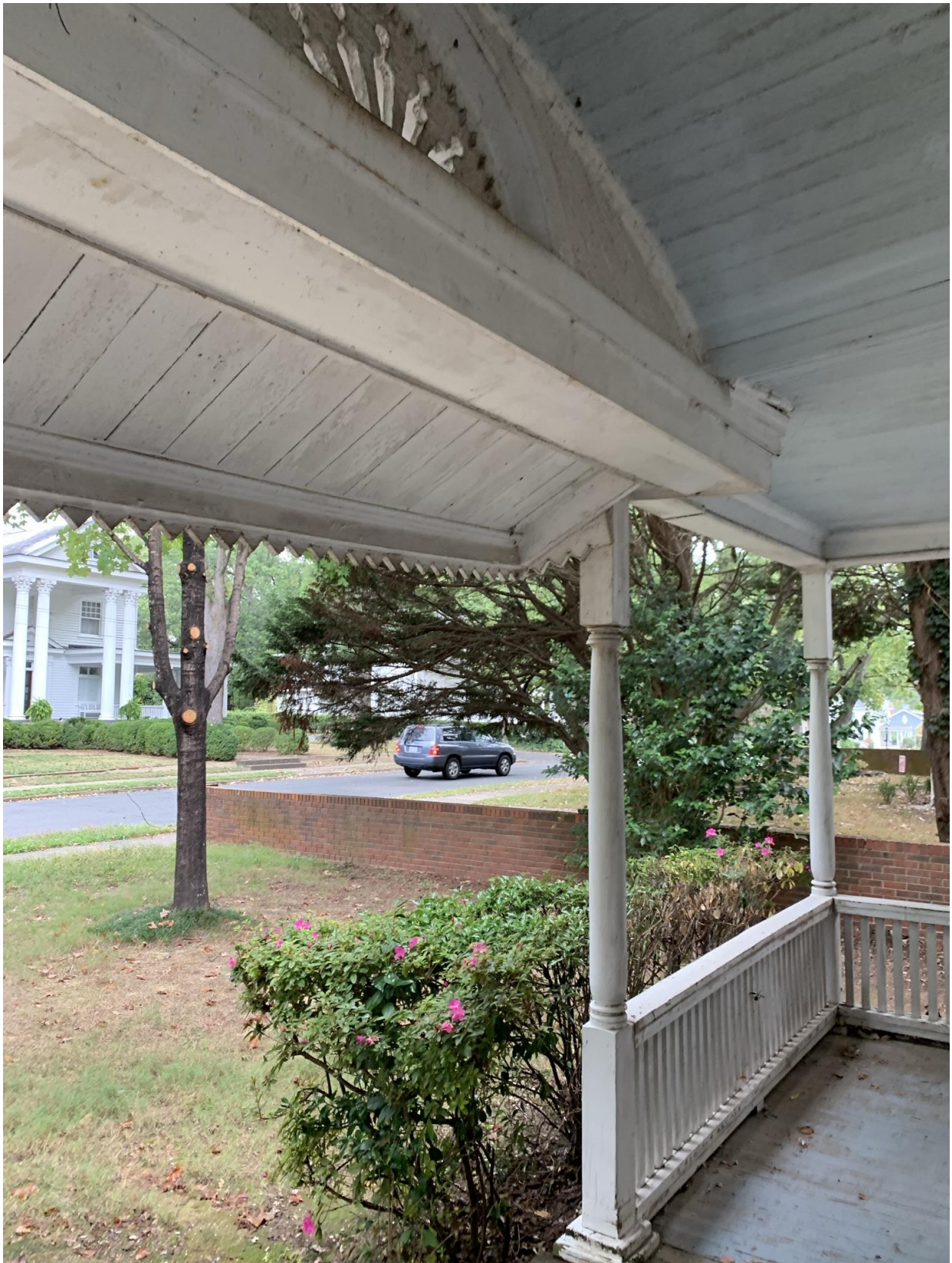
Existing columns on front porch
