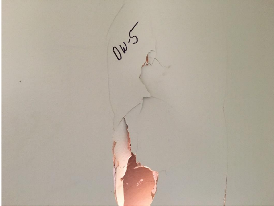
Photo 9 Structure 1; (Parcel 09-301-226B); DW-5 sample location
