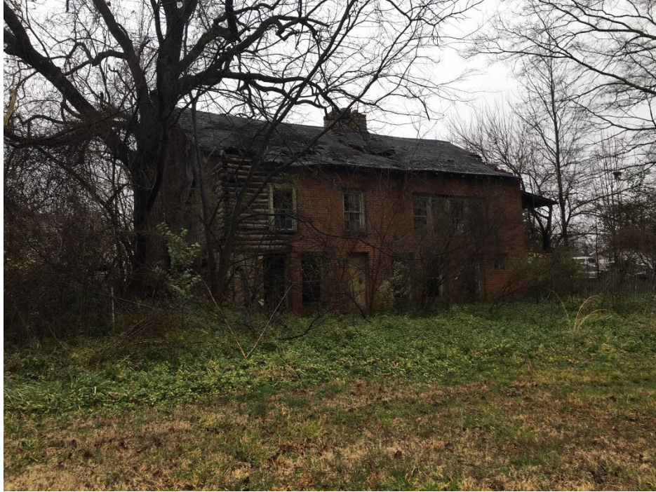
Photo 5 Abandoned structure located on Parcel 09-301-225B
