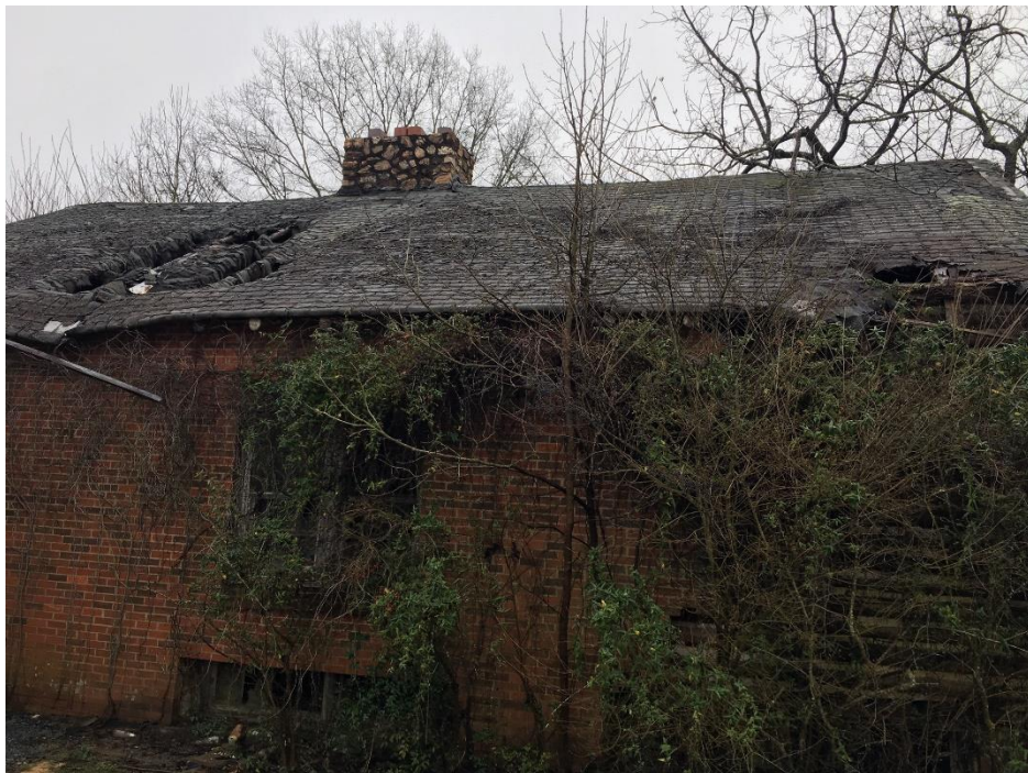
Photo 12 Exterior view of abandoned structure located on Parcel 09-301-225B
