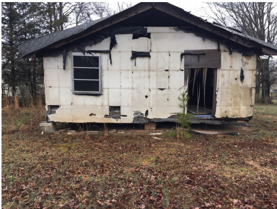
Photo 18 Abandoned structure located on Parcel 09-301-226B
