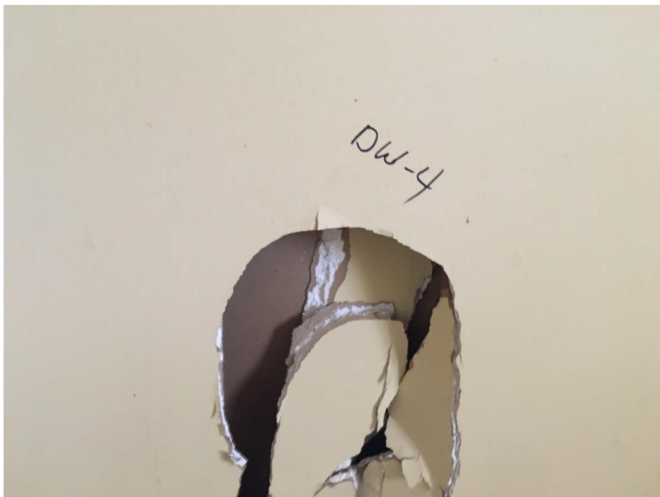
Photo 8 Structure 1; (Parcel 09-301-226B); DW-4 sample location
