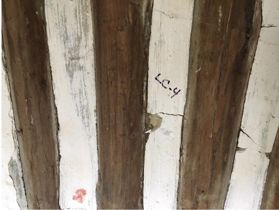
Photo 5 Structure 2 (Parcel 09-301-225B); LC-4 sample location
