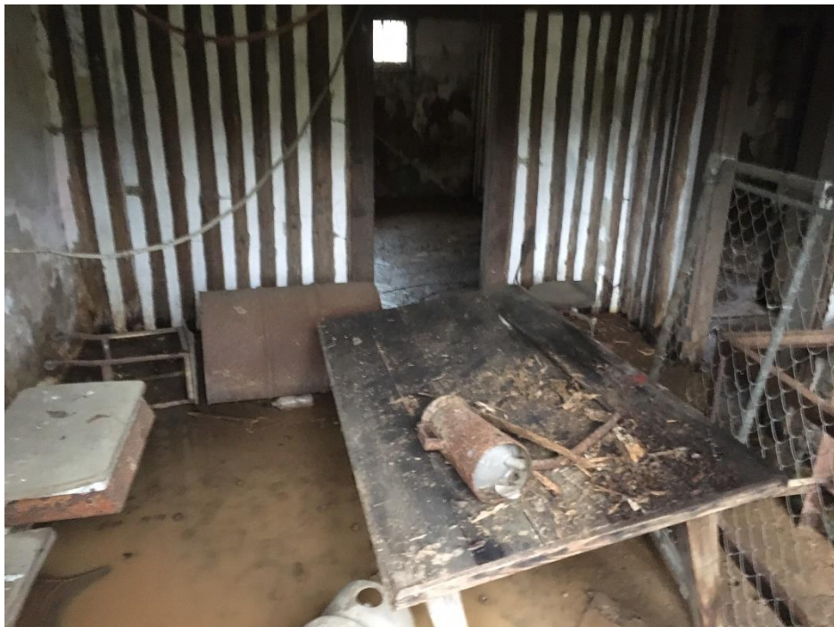
Photo 6 Interior of the basement area of abandoned structure located on Parcel 09-301-225B
