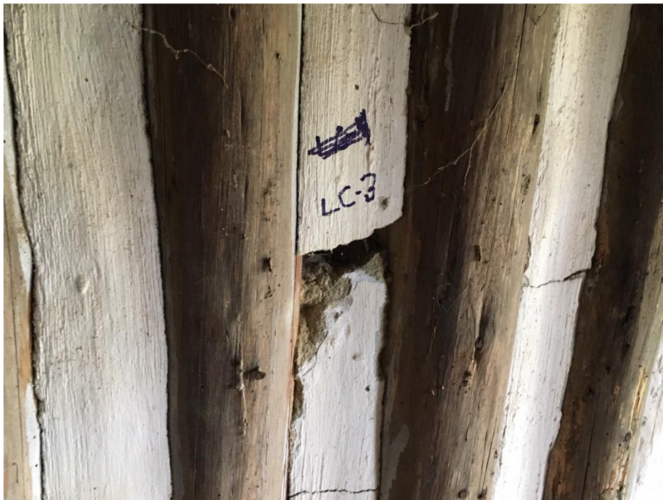
Photo 4 Structure 2 (Parcel 09-301-225B); LC-3 sample location
