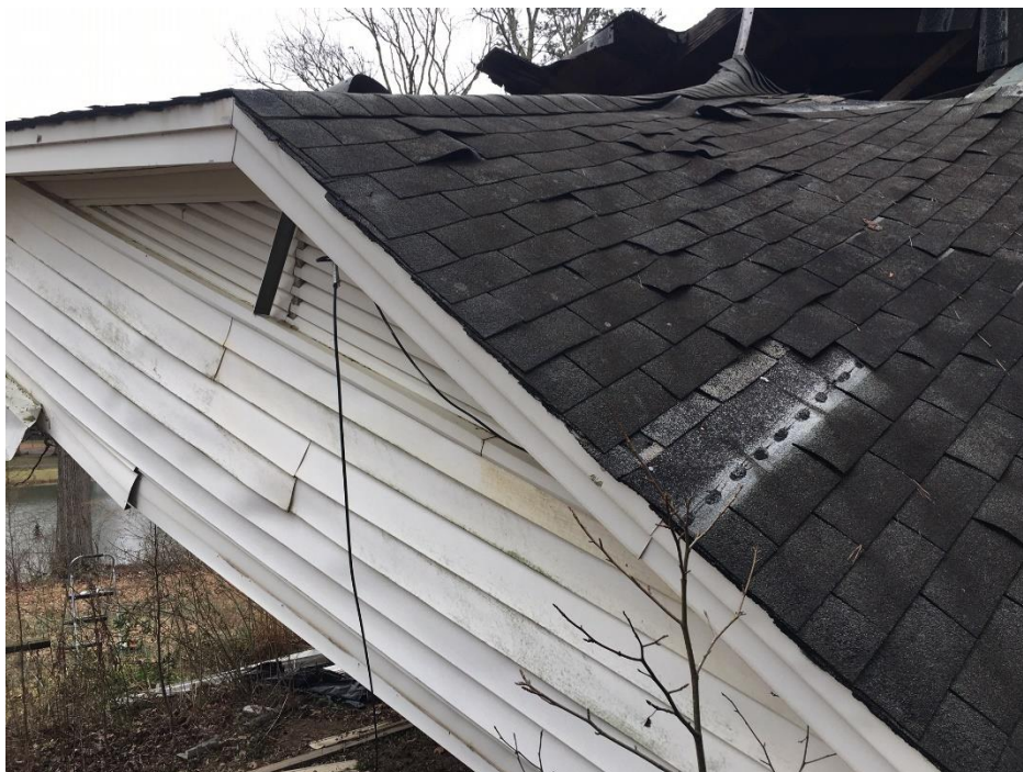
Photo 4 Structure 1; (Parcel 09-301-226B) SHIN-1 through SHIN-6 sample locations
