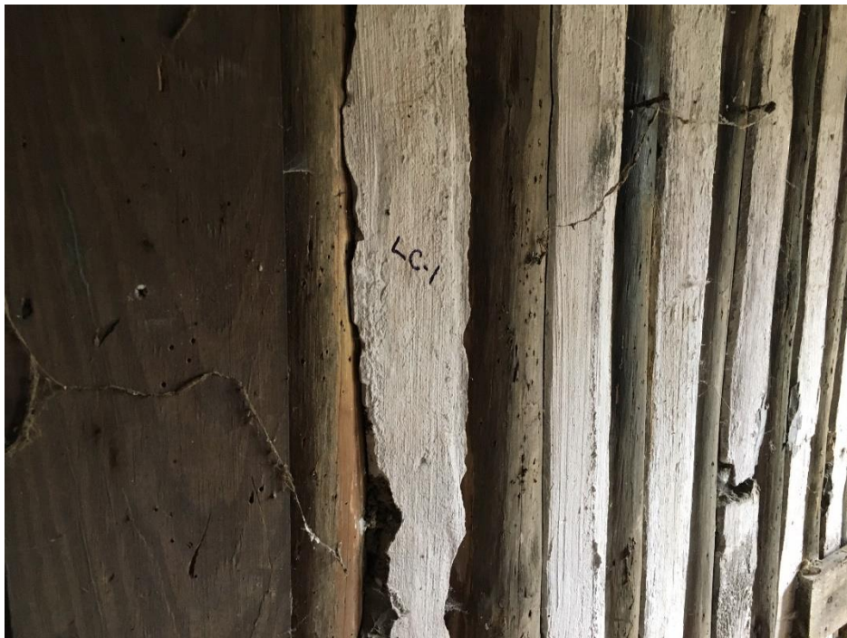
Photo 2 Structure 2 (Parcel 09-301-225B); LC-1 sample location
