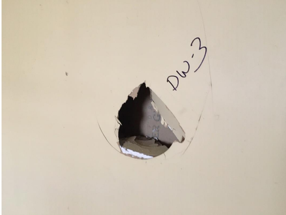
Photo 7 Structure 1; (Parcel 09-301-226B); DW-3 sample location
