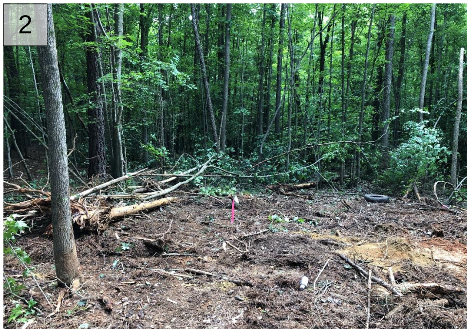
Photo 2. View of recent clearing to conduct geotechnical explorations.
